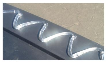
**To install:** Gel is applied in a zig-zag pattern about 3" (7.62 cm) high leaving periodic spaces for water drainage. Do not install on a vertical surface.
